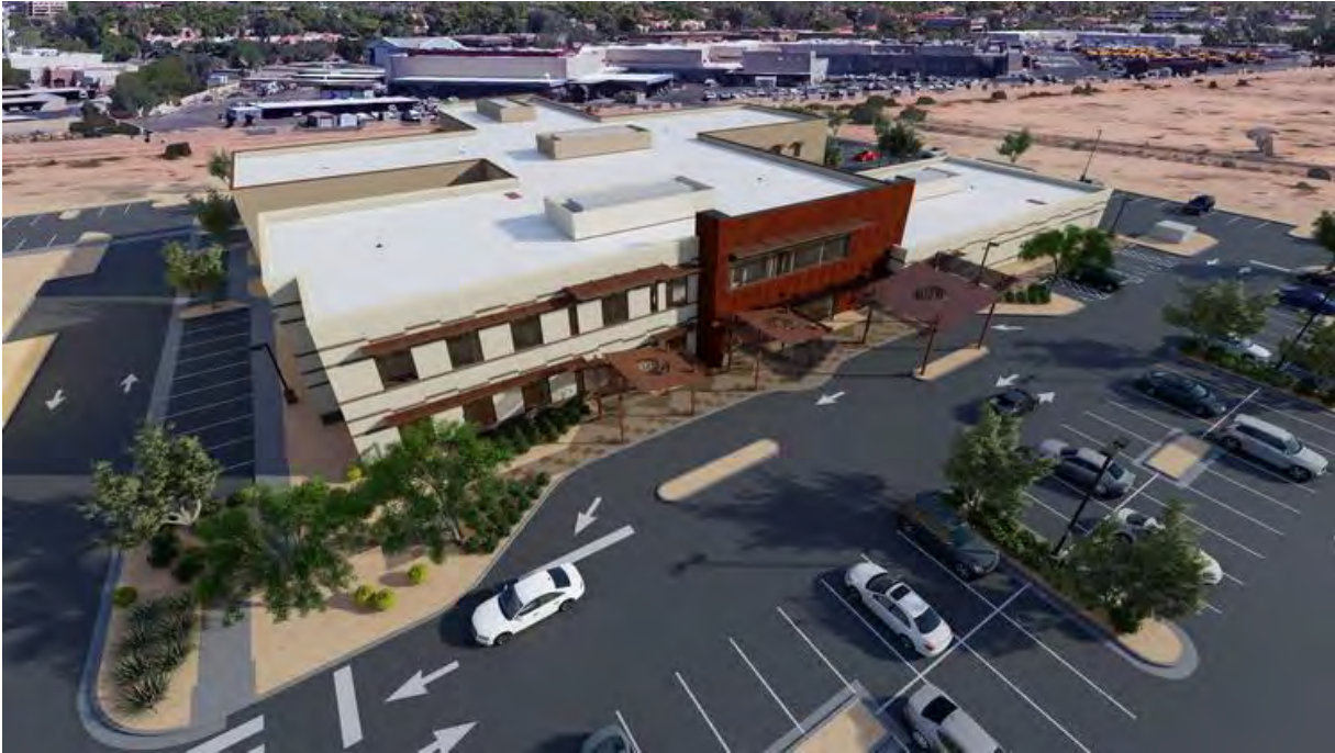
HonorHealth is teaming up with the nation's largest behavioral health system to build a hospital in Scottsdale. PROVIDED BY HONORHEALTH
